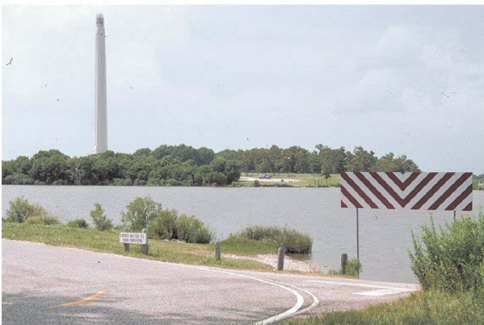
A road that provided access to the San Jacinto Monument was closed due to flooding caused by subsidence.
